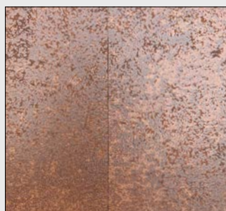
Processing without expansion gaps
